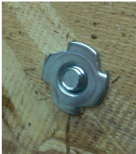
Figure 2: View from underneath the base flooring: a bolt screwed into a hammered in T- nut.
