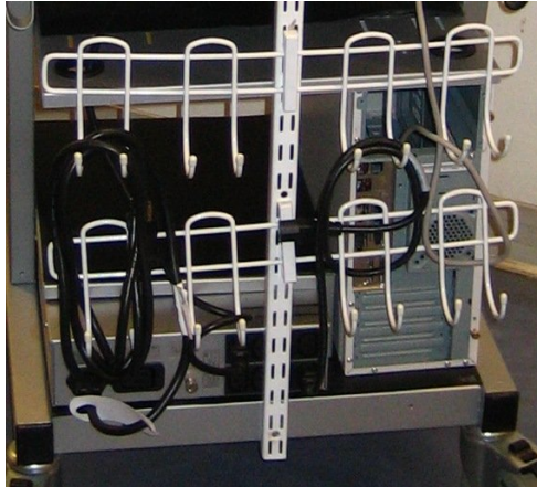
Figure XXV: The racking system shown is mounted to the back of the cart. The cables can be wound and organized on the hooks.
