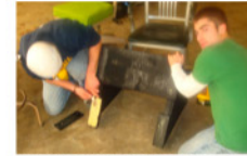
Figure 9: Fabrication of support system
