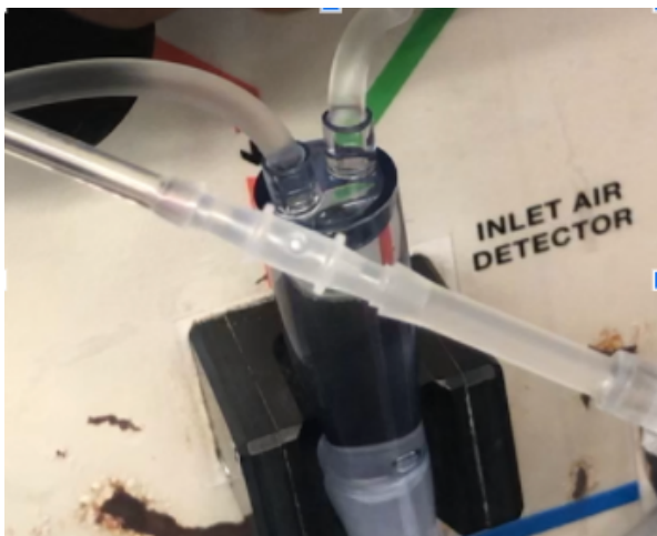
Figure 3: Close-up of tubing connectors (There is currently saline running through the joint)
