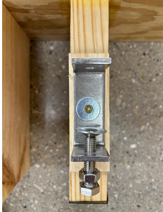
Figure [14] C-Clamp Installation
