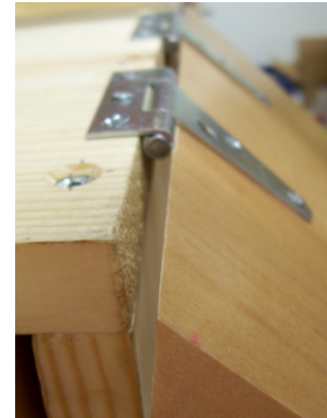
Figure 7: Hinges between headboard and wooden frame.
