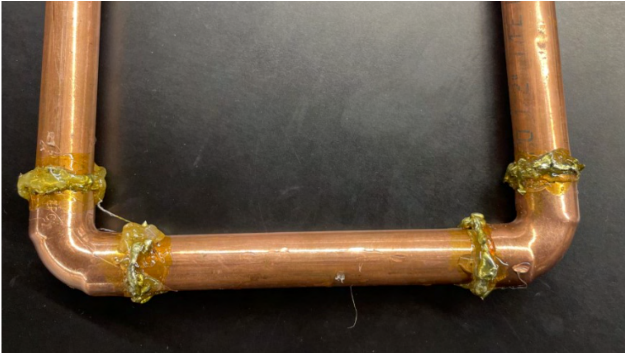
Figure 1: Photo of faulty hot glue, super glue, and electrical solder joints.
